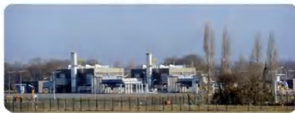
Station de compression de Nozay
